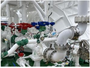
${\boldsymbol \cdot}$  Manifold onboard "EXCOOL"  $Transferring \ the \ liquefied \ CO_2 \ by \ connecting \ the \\ loading arm \ and \ ship.$
