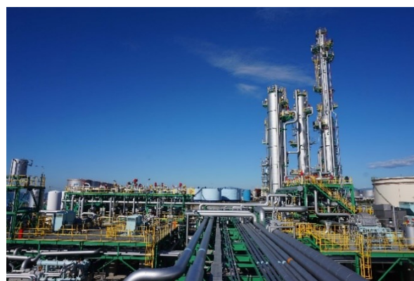
Tomakomai CCS Demonstration Project Center
